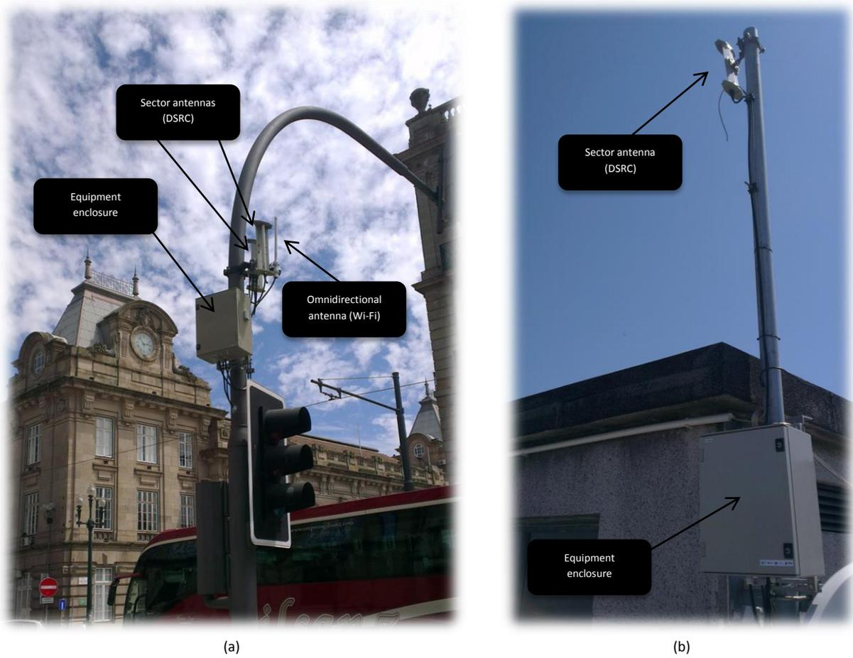
**Figure 3.2** – Examples of the road side units installed at the city of Porto: RSU3: Avenida dos Aliados is installed at a traffic light pole (a) and RSU5: Câmara Municipal do Porto (Trindade) is installed at a public building (b).
